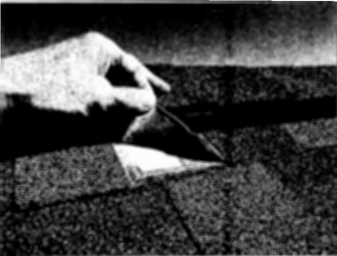
Photo 4 depicting delamination in Shingles.
